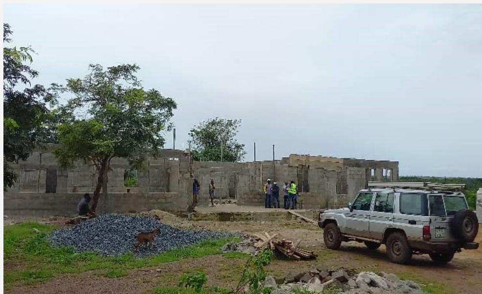
One of NaCSA CDDP subproject under construction
