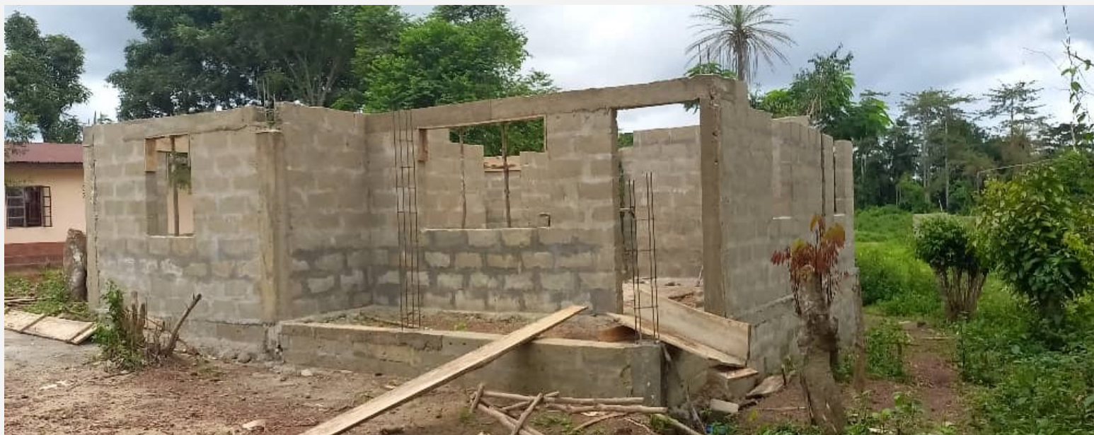
Another subproject under construction by the NaCSA CDDP Programme
