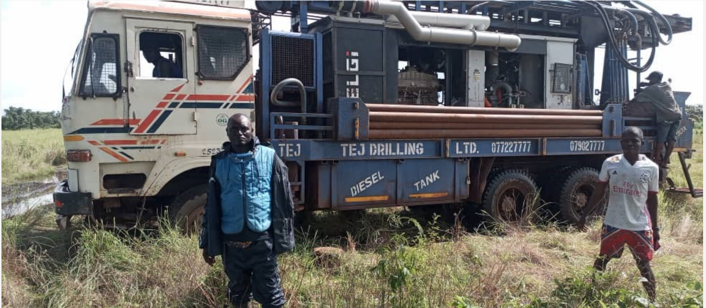
Drilling operators at work in one of the communities in Kambia District
